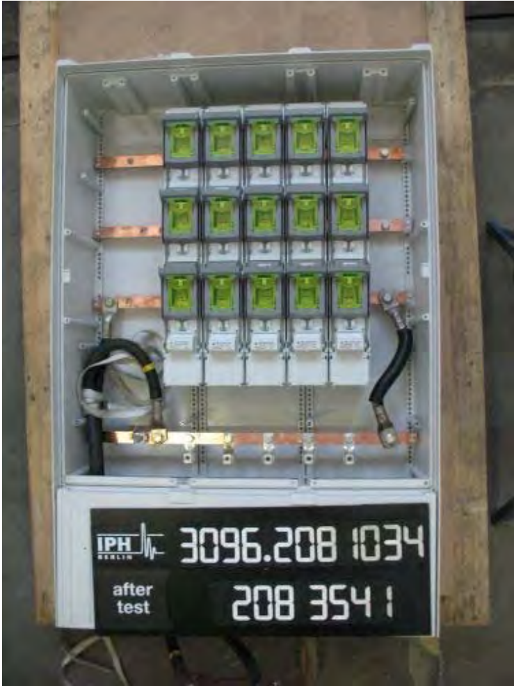
Photograph 7: Arrangement for the short-circuit test of the PEN bar (Condition of test object after short-circuit test)
