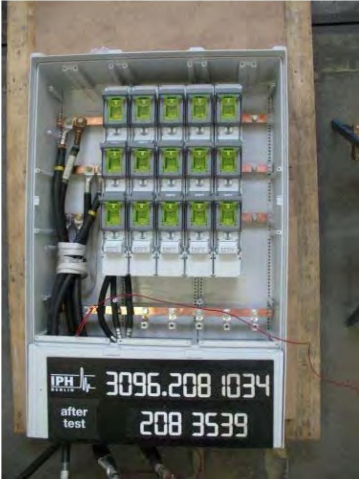
Photograph 6: Arrangement for the short-circuit test of the outgoing circuit no. 1 (Condition of test object after short-circuit test)
