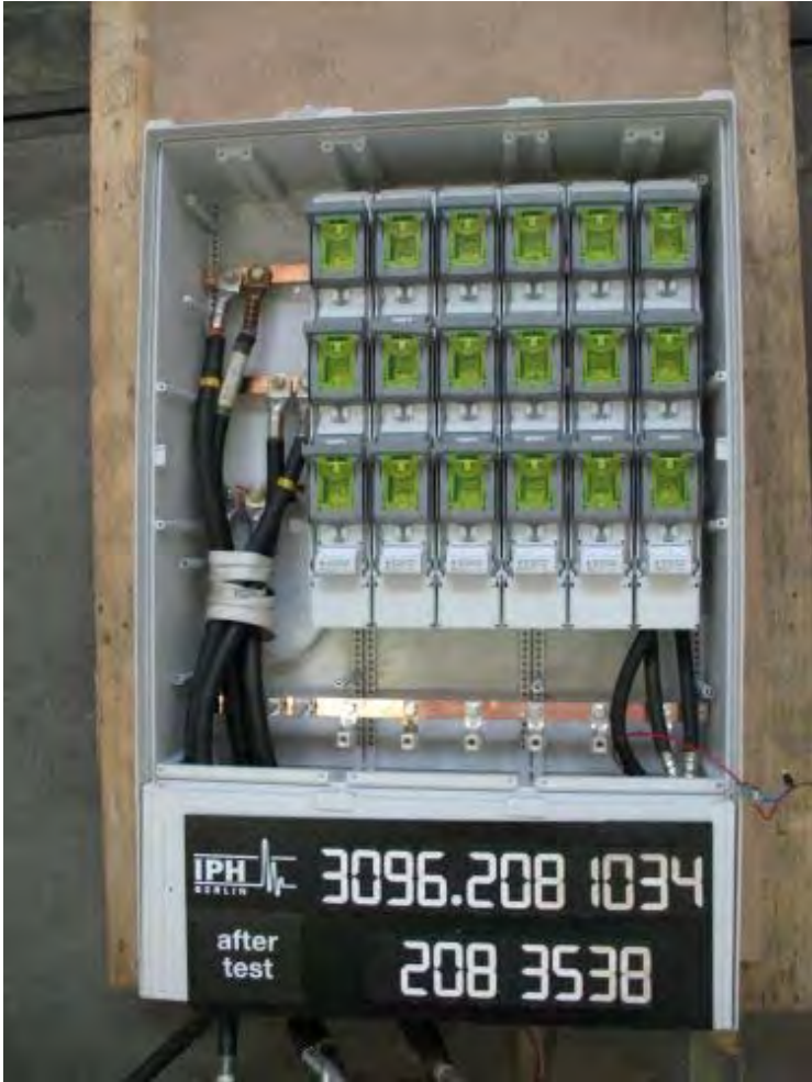
Photograph 5: Arrangement for the short-circuit test of the outgoing circuit no. 6 (Condition of test object after short-circuit test)
