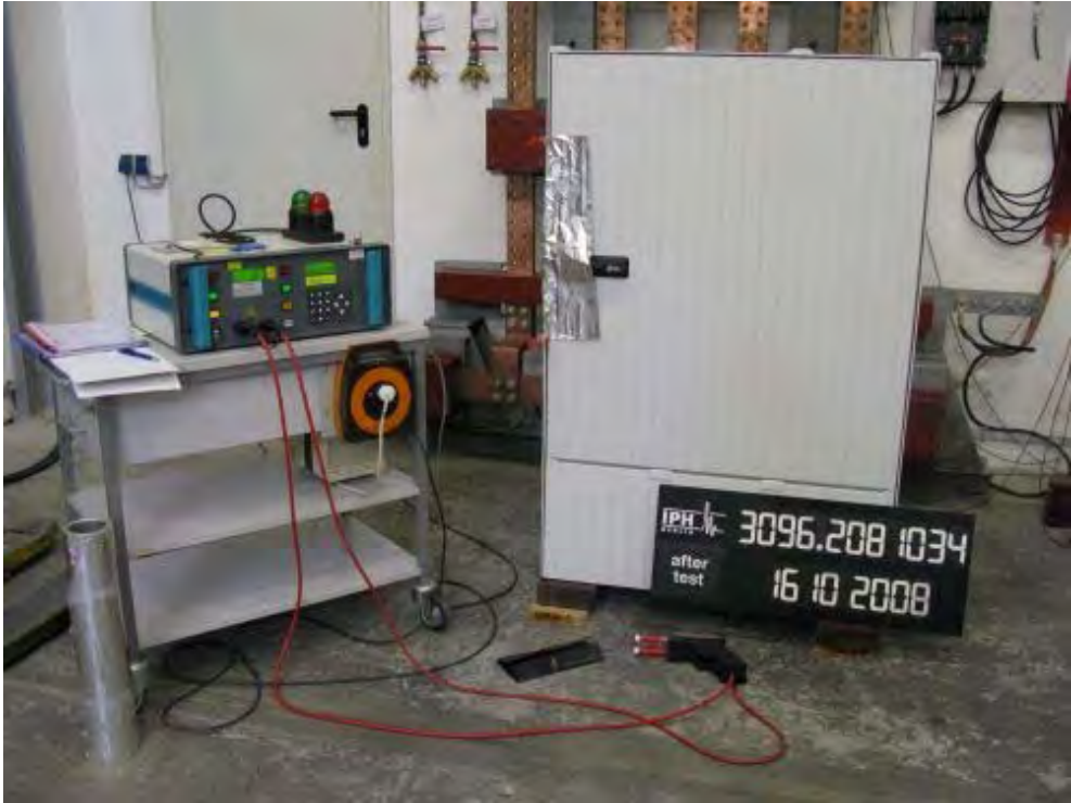
Photograph 8: Arrangement for voltage test
