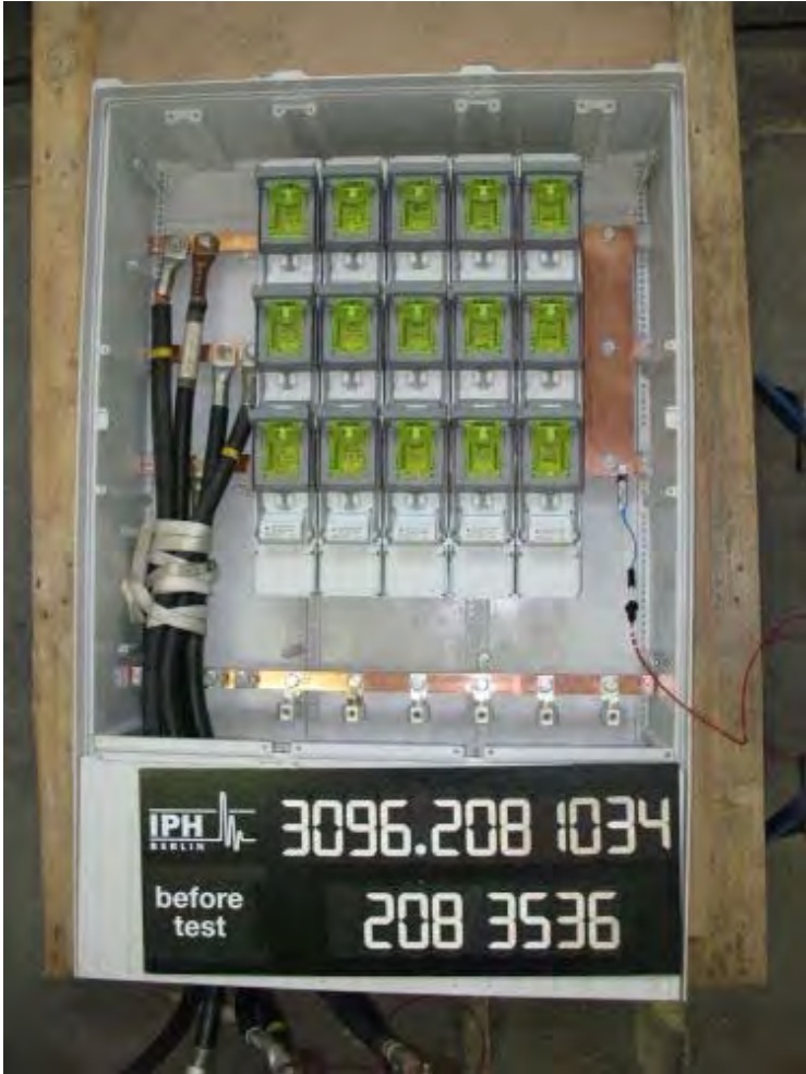
Photograph 3: Arrangement for the short-circuit test of the main busbars (Condition of test object before short-circuit test)
