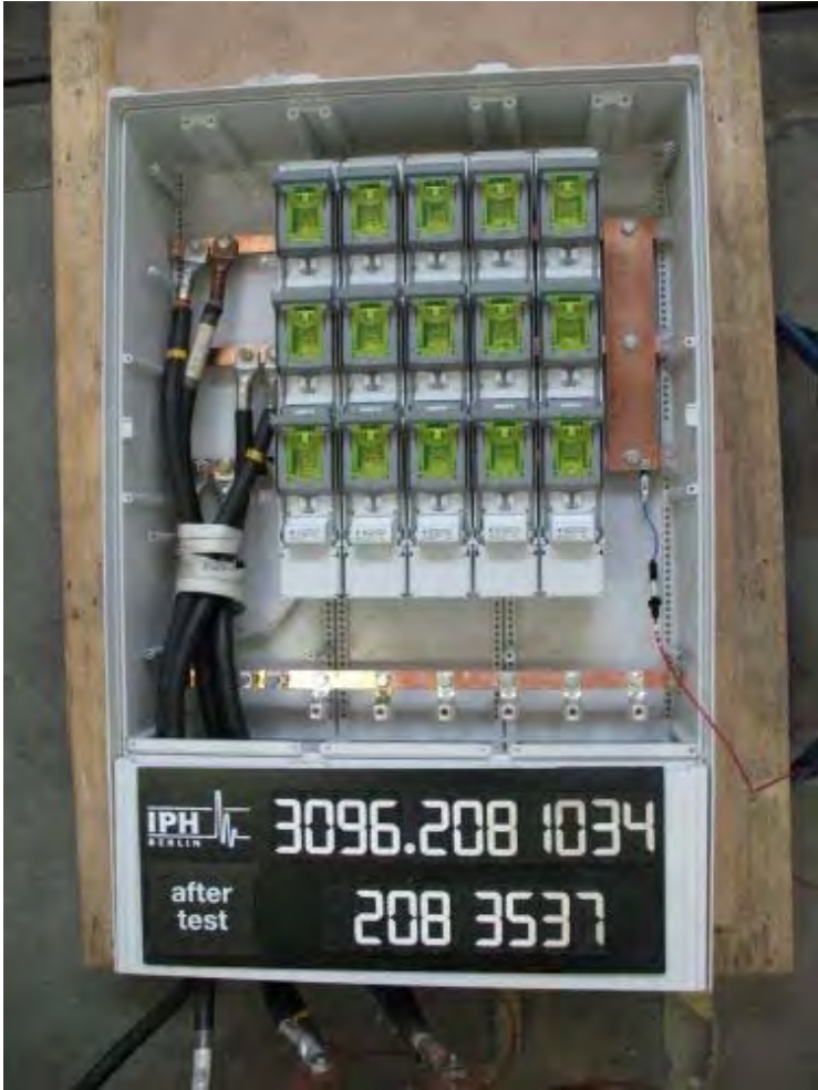
Photograph 4: Arrangement for the short-circuit test of the main busbars (Condition of test object after short-circuit test)
