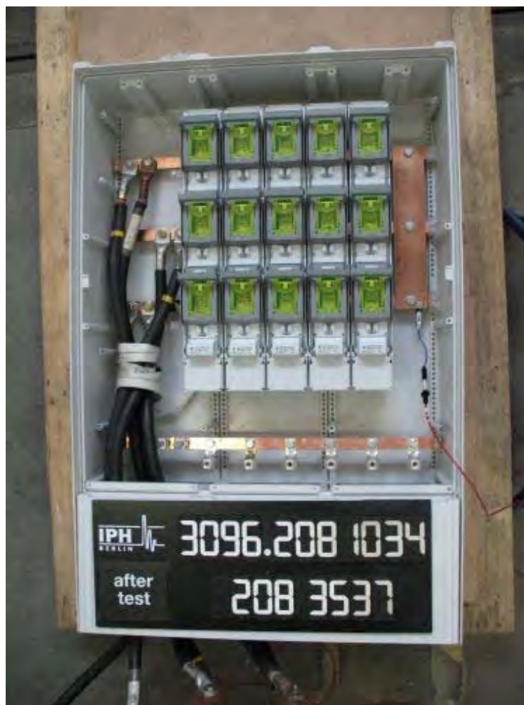
Photo 4: Arrangement for the short-circuit test of the main busbars (Condition of test object after short-circuit test)
