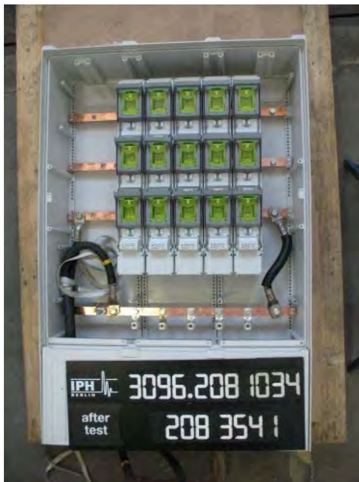
Photo 7: Arrangement for the short-circuit test of the neutral bar (Condition of test object after short-circuit test)
