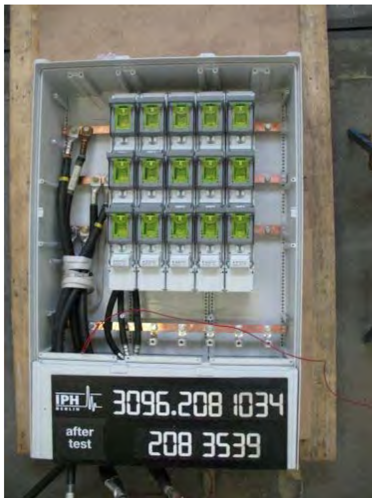
Photo 6: Arrangement for the short-circuit test of the outgoing circuit no. 1 (Condition of test object after short-circuit test)
