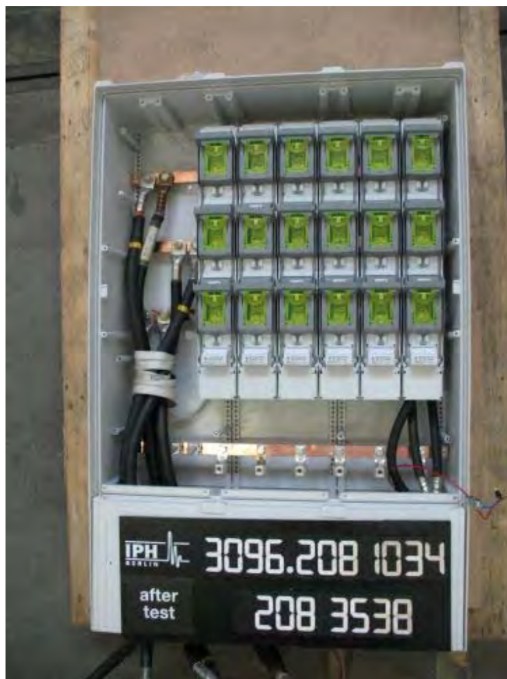
Photo 5: Arrangement for the short-circuit test of the outgoing circuit no. 6 (Condition of test object after short-circuit test)
